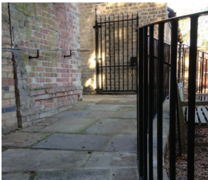
The new ramp en route to Brookside
