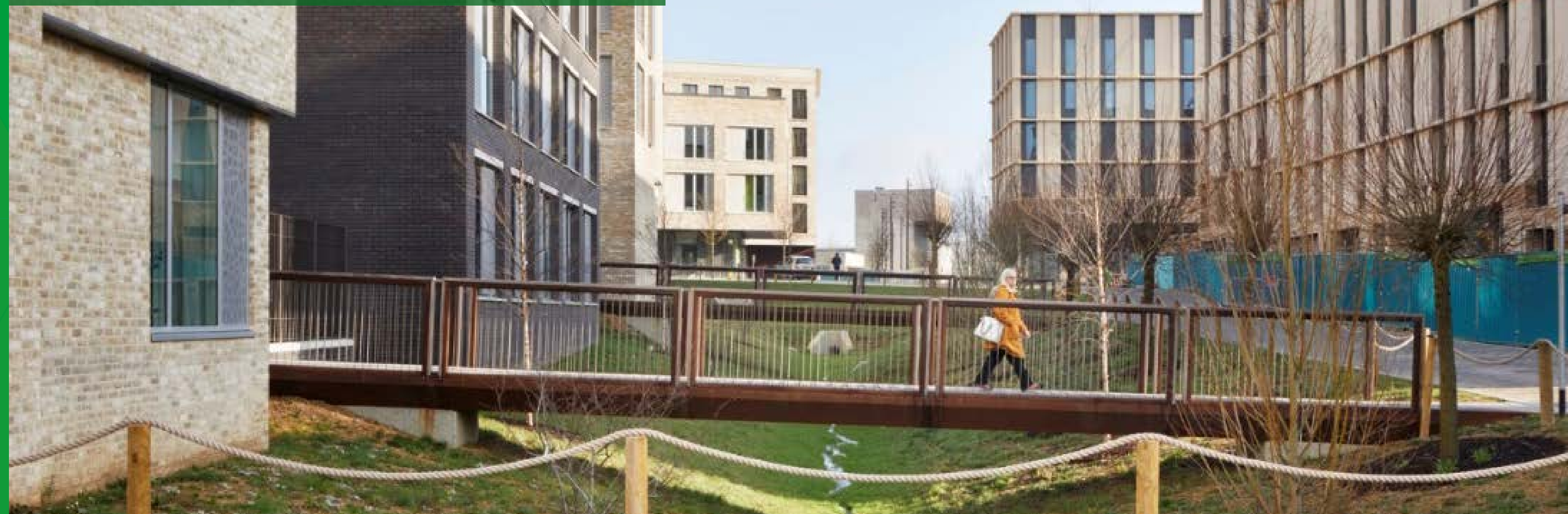
Swale enables the surface water to drain to the lakes as part of the Sustainable Urban Drainage System
